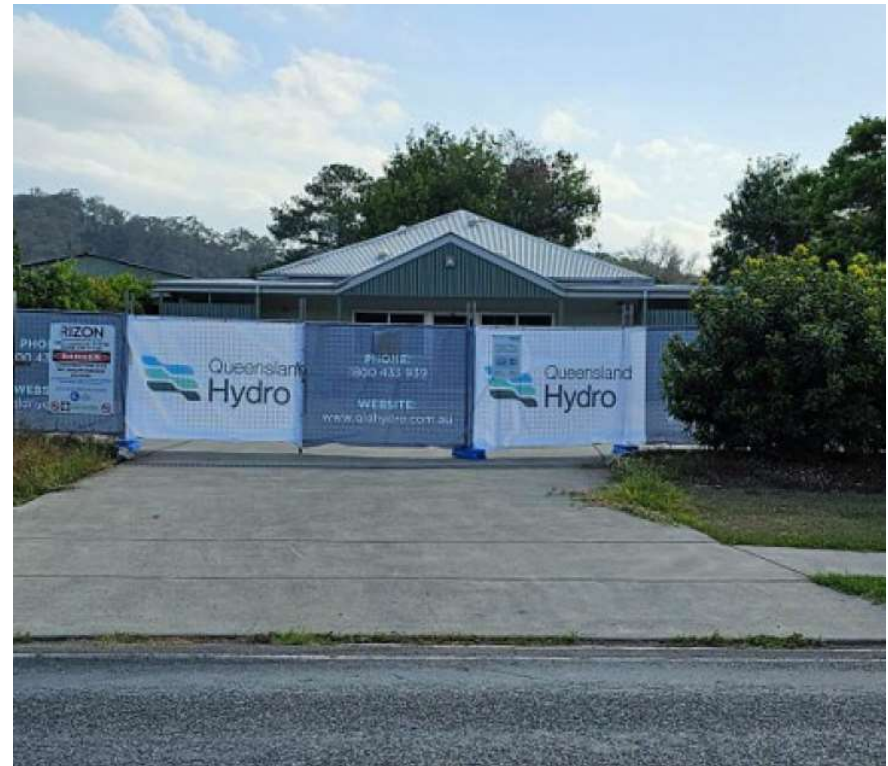
Queensland Hydro Imbil Office anticipated to open in December 2023. Office hours are yet to be determined.
