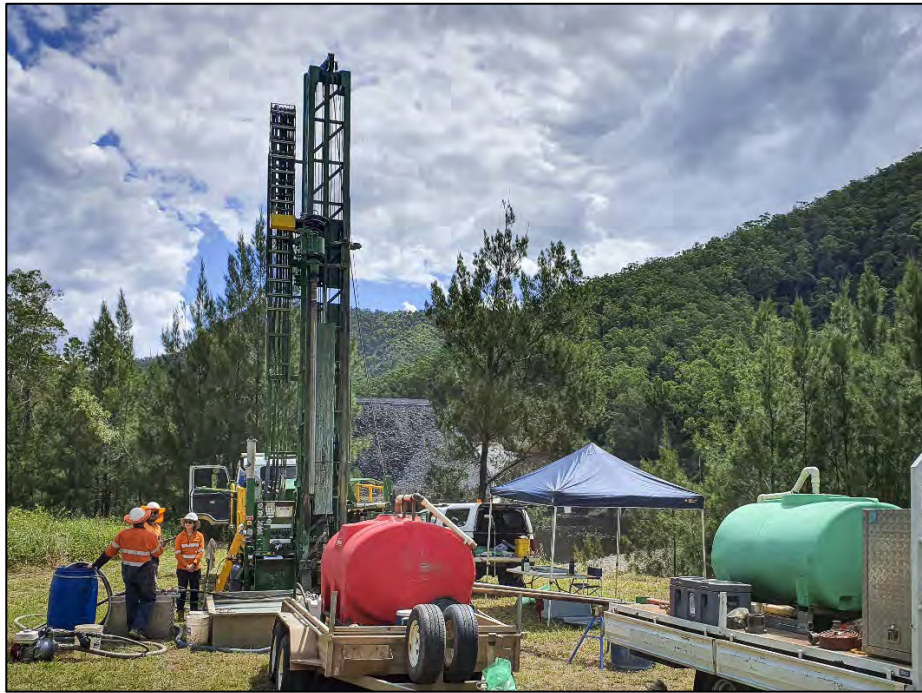
Figure 3-2 Geotechnical drill rig
