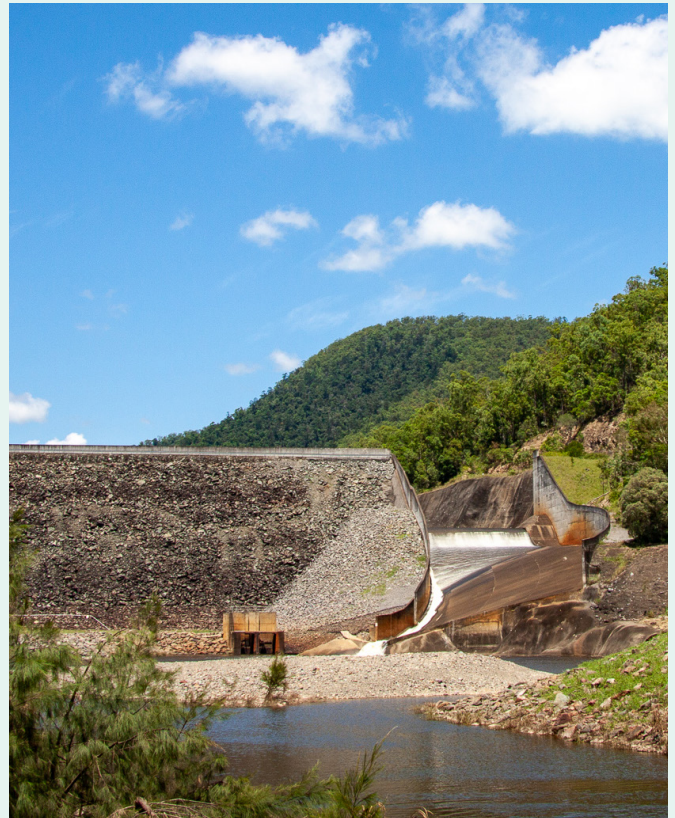
The existing Borumba Dam
