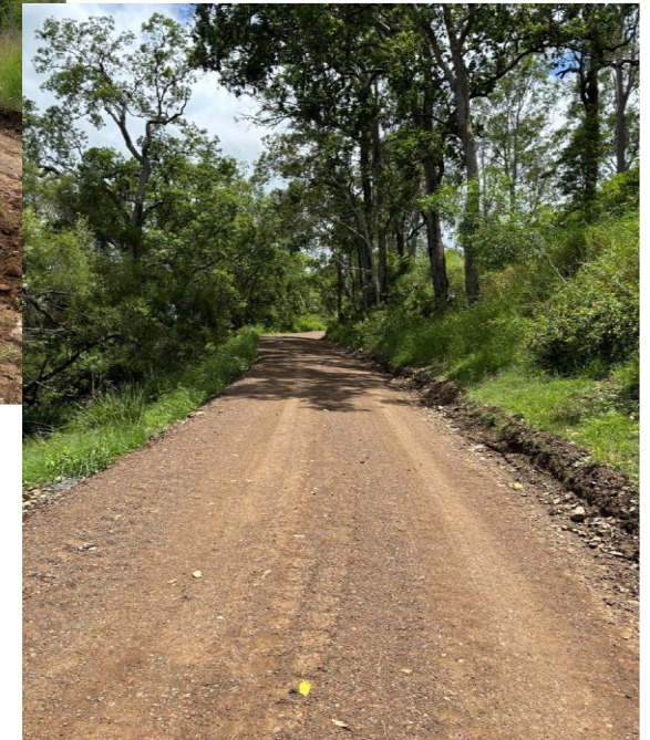
Earthland Group started the Borgan Road Re-sheeting process in January 2024.
