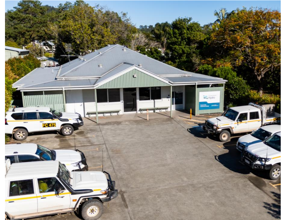
GP Clinic and Queensland Hydro Office, 6 Imbil Island Road
