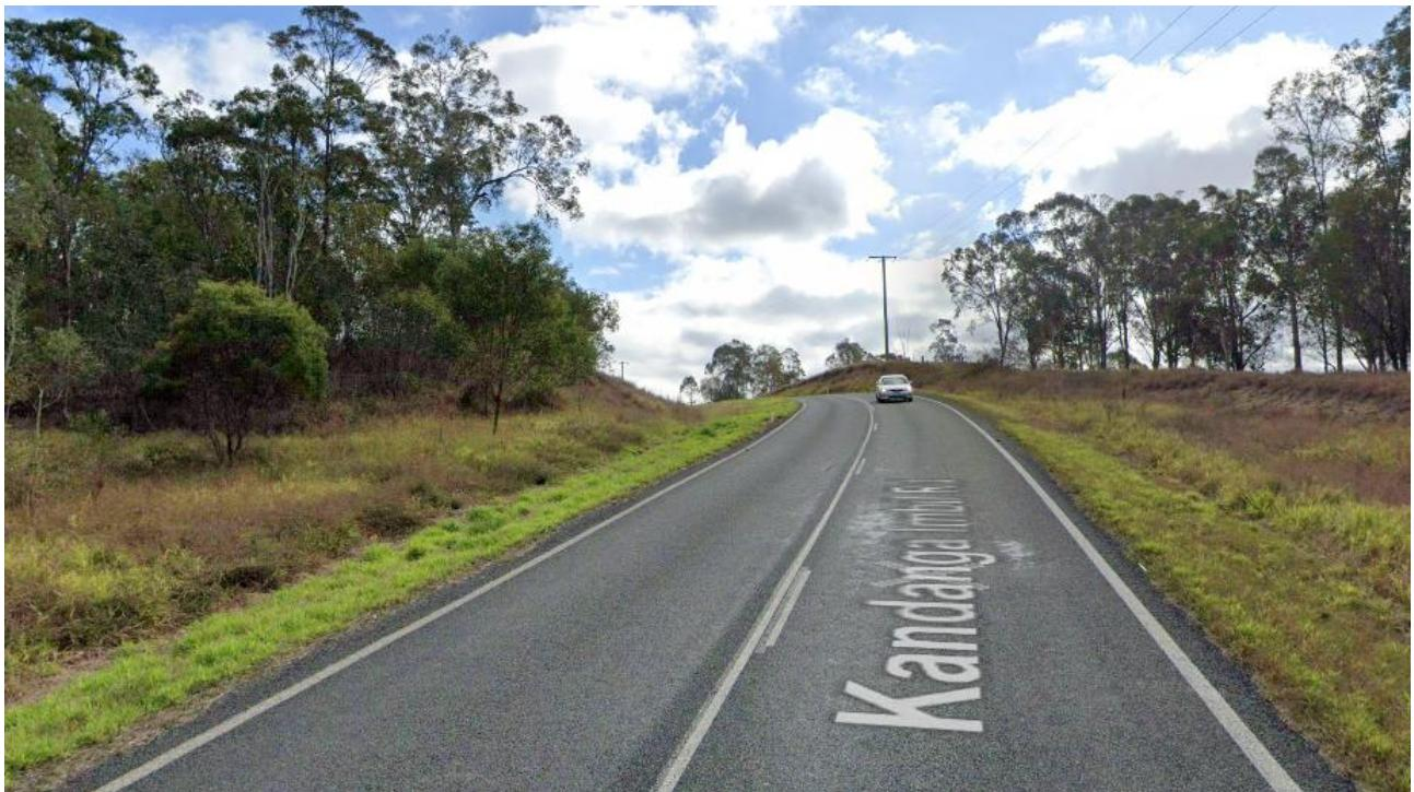
Figure 3–6: Kandanga Imbil Road (CH 20.5 km) – note combination of vertical and horizontal changes in alignment reducing sight lines.
