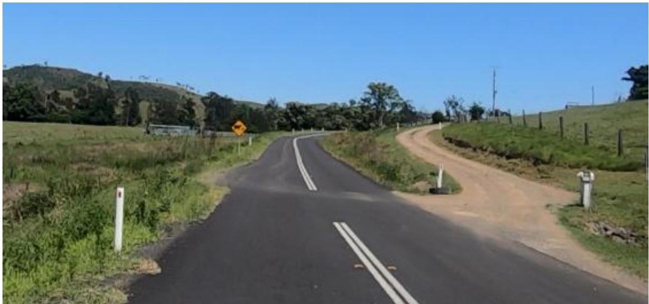
Figure 3–28: Kilcoy Murgon Road / Ten Mile Road intersection with poor approach sight lines due to changing alignment
