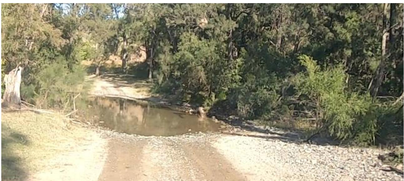
Figure 3-21: Bella Creek Road – example of water crossing and trees restricting ability for opposing vehicles to pass
