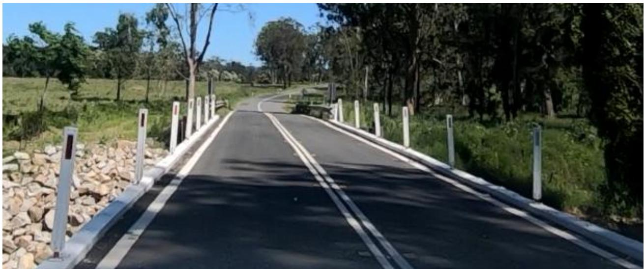
Figure 3–27: Kilcoy Murgon Road – Sheep Station Creek 2 bridge crossing – Narrow Road width, no shoulders, no safety barriers
