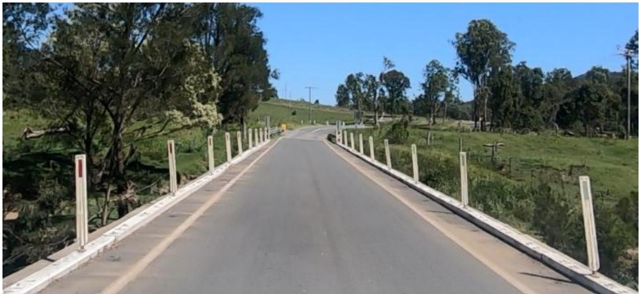
Figure 3–26: Kilcoy Murgon Road – Sheep Station Creek bridge crossing – single lane and no safety barriers
